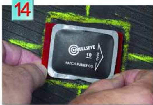
**14.** When cement is dry, partially remove the poly backing from the patch leaving just enough to hold the patch. Do not touch the back of the patch. With the beads of the tire in the relaxed position, apply the patch to the buffed area making sure the bead arrow points to the bead. Remove the remaining poly from under the patch.
